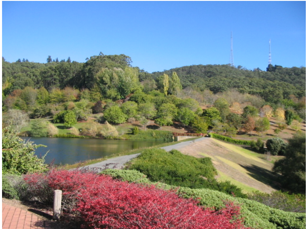
Figure 8.1 Photograph of the Main Dam embankment looking north-north-west towards Mount Lofty summit. Source: David Jones
